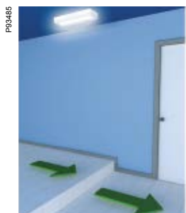
Near every change in floor level.
